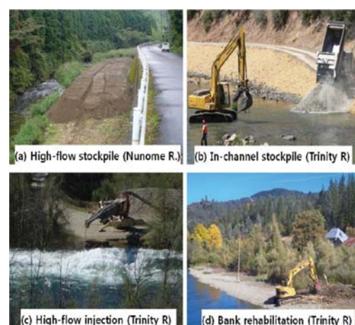
Figure 1. Sediment augmentation methods depending on implementation techniques.
