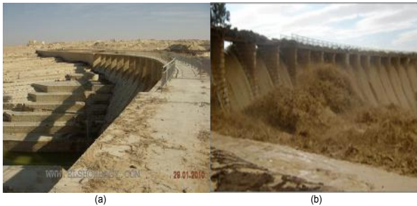
Figure 6. El-Rawafaa Dam before the flash flood (a), and during the flash flood event of Jan, 2010, showing how much of the water is overflowing the dam
