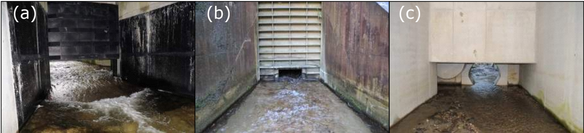
Figure 3: Bottom outlet design: (a) Lafiniz-Waldbach, (b) Ligistbach and (c) Labuchbach.
