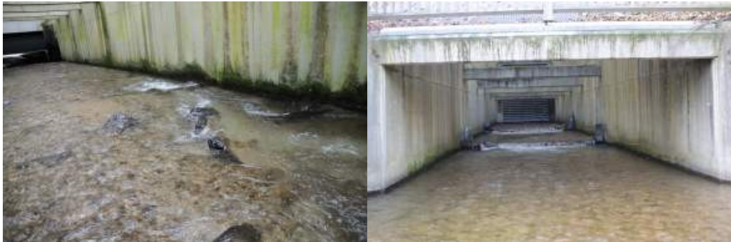
Figure 6: Bottom outlet design for fish passage by using natural stones and stepped pools
