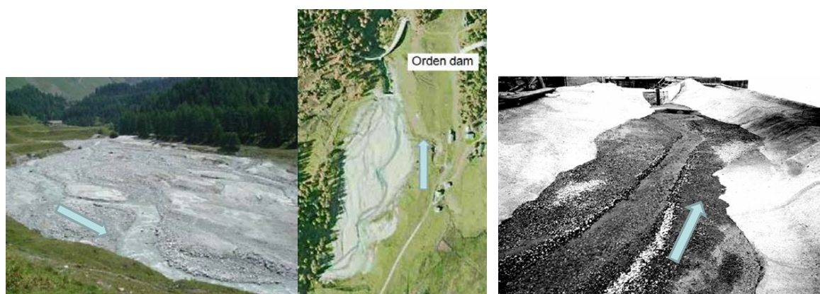
Figure 8 Reservoir sedimentation of Orden dam in Switzerland (Left: From dam to upstream view, Middle: Aerial view, Right: From upstream to dam on the model study)
