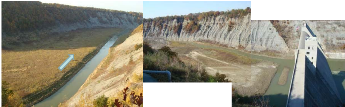
Figure 9 Reservoir sedimentation of Mount Morris dam in USACE Buffalo District (Left: Channel erosion, Right: Sediment deposited just upstream of dam is periodically dredged)
