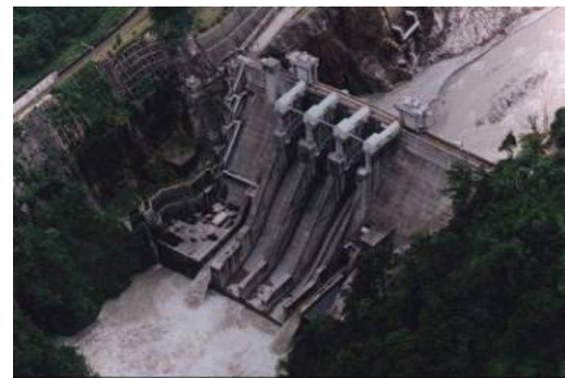
Fig. 4 Aerial photo from free-flow sediment flushing at Dashidaira Reservoir.
