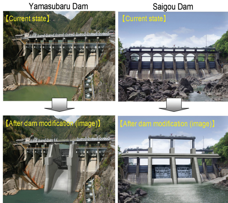
Above: Figure 3 – Case studies for dam retrofitting works on Yamasubaru and Saigou Dams (Sumi et al., 2015)
