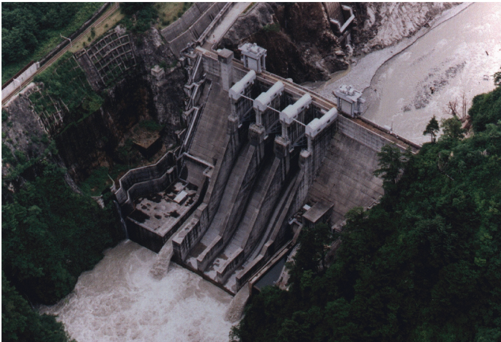
Figure 14.8 Photographs of (a) Unazuki and (b) Dashidaira dams during coordinated sediment flushing operation (Sumi et al. 2009).
