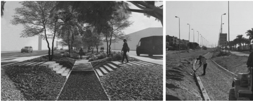
Fig. 11.25 Bioswales, storm planters, and infiltration tools in New Cairo city
