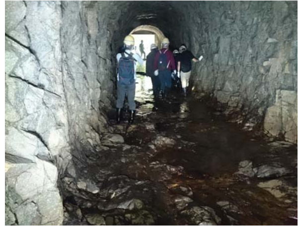
Unlined tunnel of Nunobiki-Gohonmatsu constructed more than 100 year ago.
